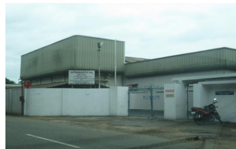
Fig 10.A.1 Existing coir industries in town
